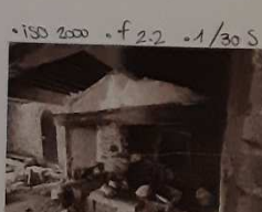
I used this photo because I thought that this room was burnt and so, it gave me at the same time, sadness.
